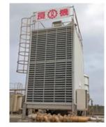
The Dayuan factory completed the addition of an LCC-S type water-saving closed-loop cooling tower (LCC-V-125S) to the tonic beverage line.
