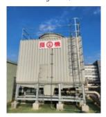
The Zhongli factory completed the installation of a 300RT energy-efficient, water-saving, and low-noise cooling water tower.
